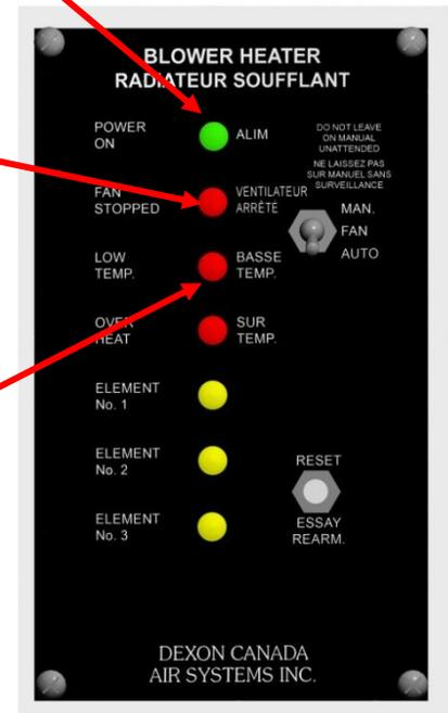
Figure 4: “Fan Stopped” Indication with “Low Temp.” Indication
