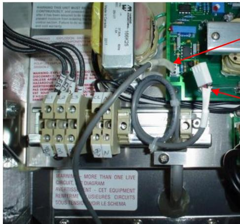
Temp. Sensor Jack with Dexon Simulator Connection
