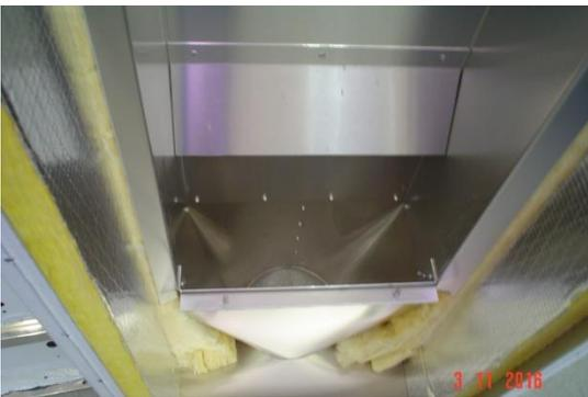
Fig. 5 – **IMPORTANT:** Plug hole to prevent gases and moisture from entering the area. **CAUTION:** This area may no longer be classified as non hazardous and confined entry procedures must be observed.
