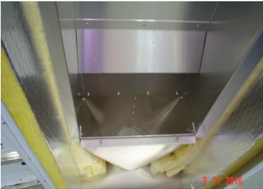
Fig.5 - **IMPORTANT:** Plug hole to prevent moisture and gases from entering the environment. **CAUTION:** This area may not longer be classified as non hazardous while the unit is down and confined entry procedures must be observed
