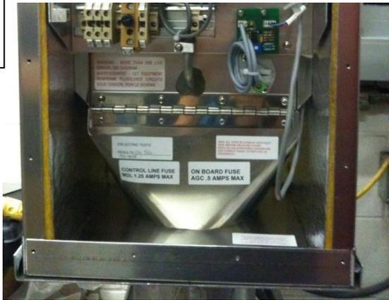
Fig.3 - Remove the insulation from the bottom section and remove screws on the hinge. Now you can remove control/element section from the transition by grasping the top of the control section with one hand and the 3/8" aluminum tube at the bottom with the other and gently pulling towards you.
