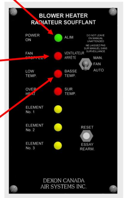
Figure 4: “Fan Stopped” with “Low Temp.” Indication
