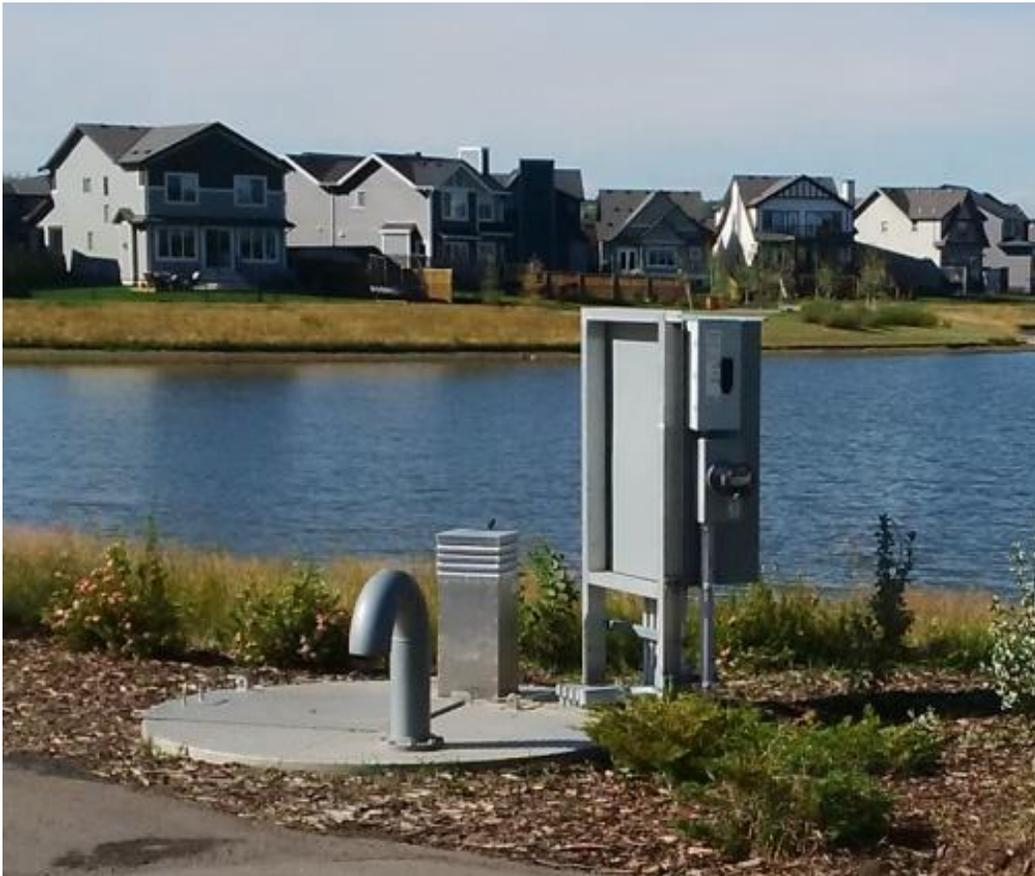
PROVIDING SAFETY VENTILATION TO THE WATER, WASTER WATER INDUSTRY
